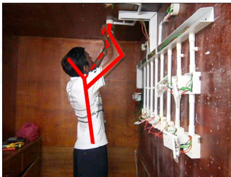
Fig. 3. Ceiling Height installation for activity 2
