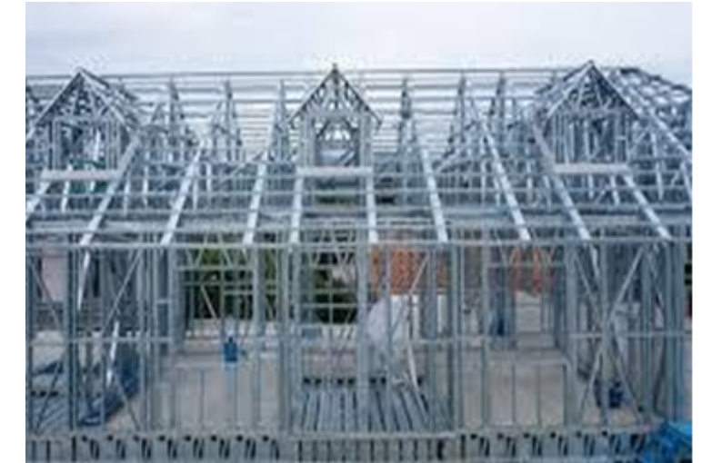
Fabricated steel structures
